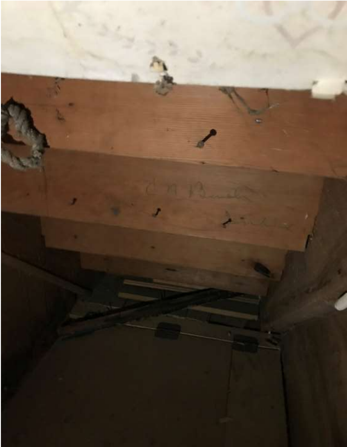
Signature of Clarence Bush in Stairwell, main floor
