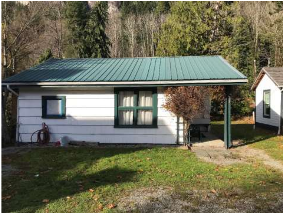
Caretakers Cottage, constructed c. 1935, (non-contributing) currently storage (view north).
