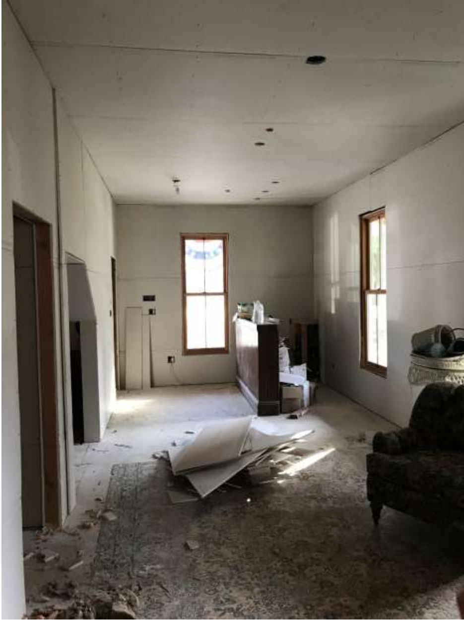
Bush House Interior, Main Floor, west side, during drywalling (view south).
