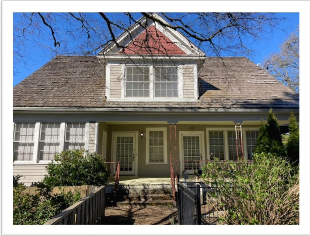
Figure 4. Sawyer House Façade (view west).
