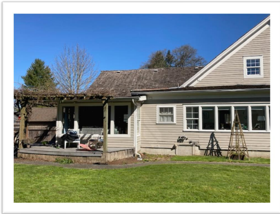
Figure 10. South side of house with deck and trellis (view northwest).
