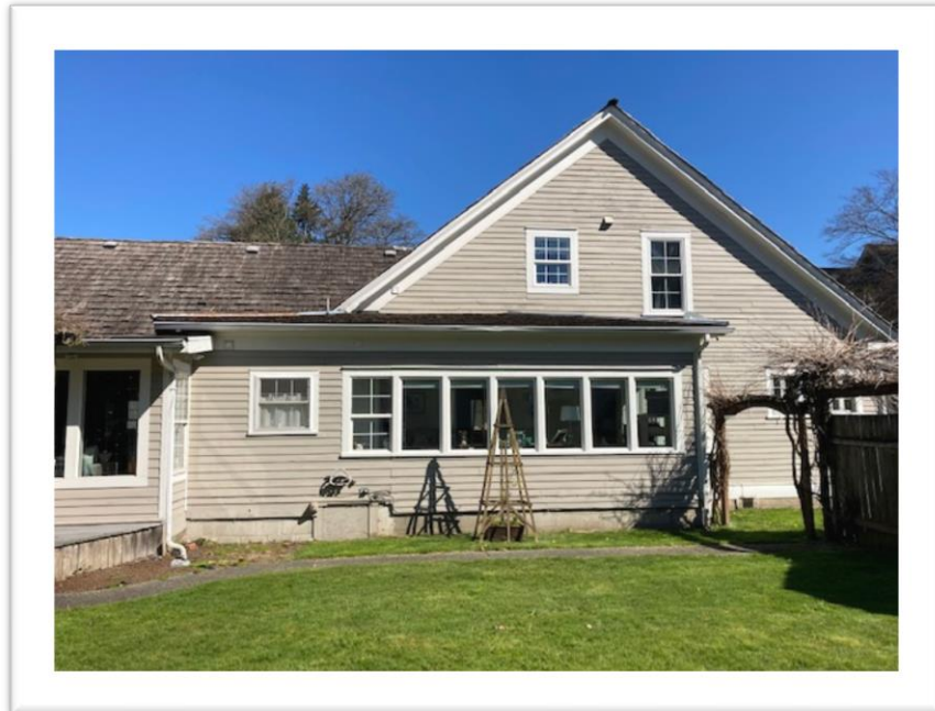
Figure 9. Sunroom addition on (view east).
