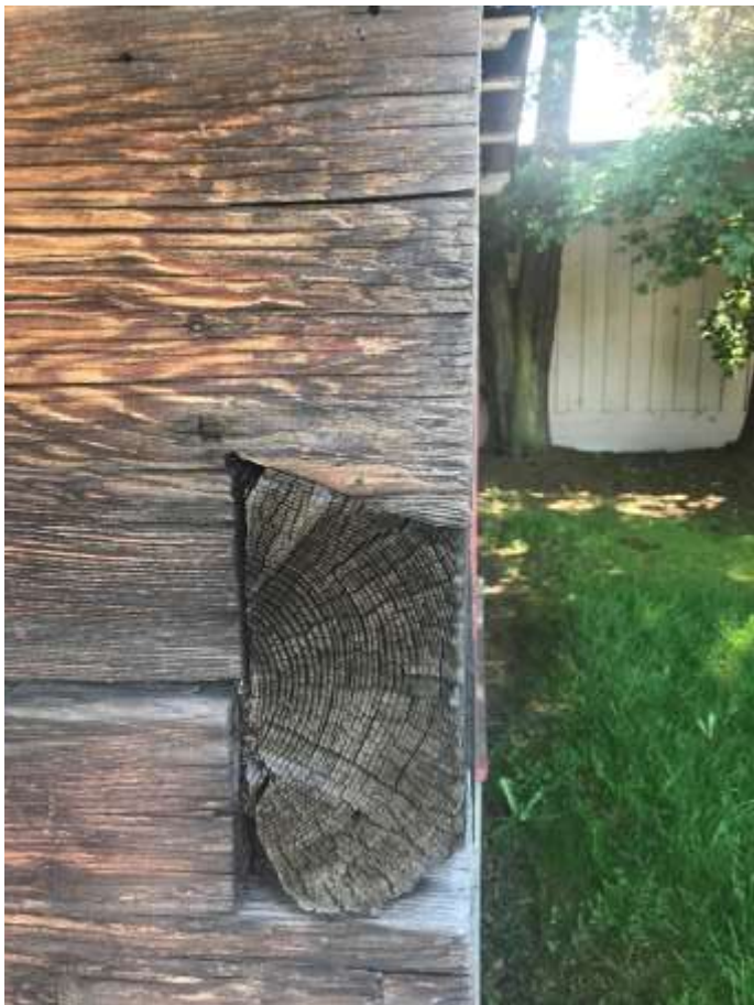
Figure 3. Half dovetail notching southwest corner
