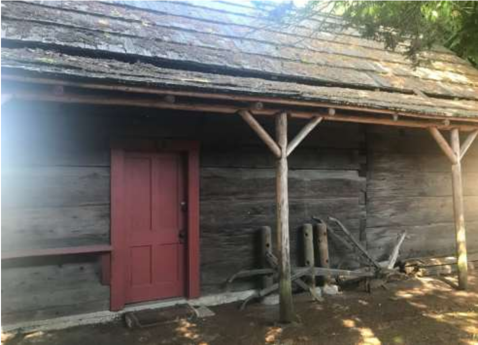
Figure 2. Shannahan Cabin east façade (view west)
