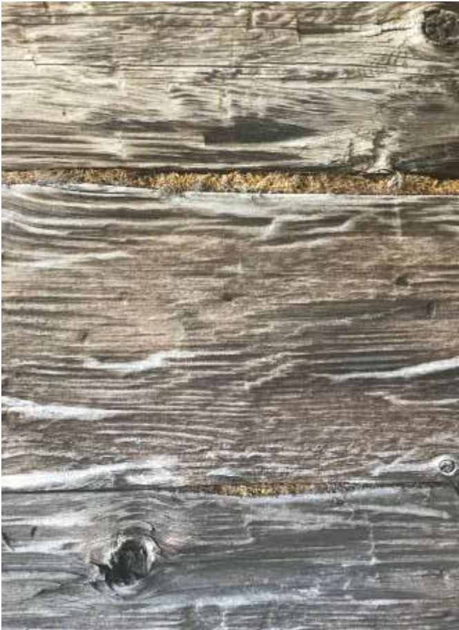
Figure 4. Hand hewn log detail (west façade)
